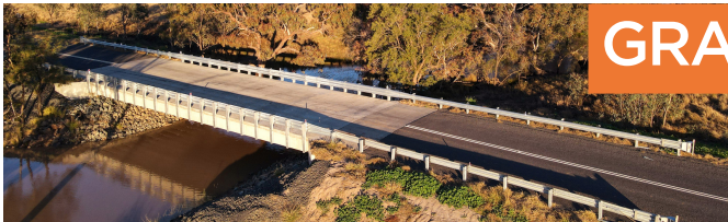
THE $1.15M UPGRADE TO WONBOBBIE BRIDGE, WONBOBBIE ROAD ON MARTHAGUY CREEK IS NOW COMPLETE Image credit: Steven Christian
