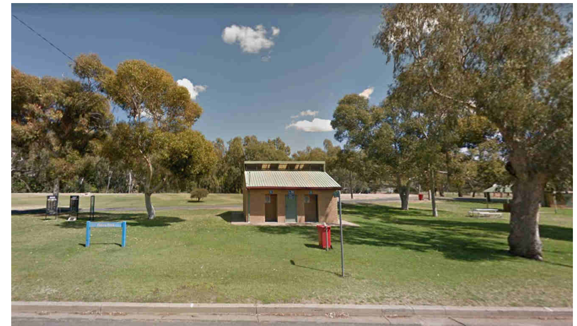
View from Oxley Hwy - Rest Area (toilets)
