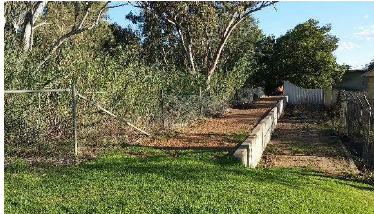
Macquarie River levee/river walk (widen / signage / gravel / safety)
