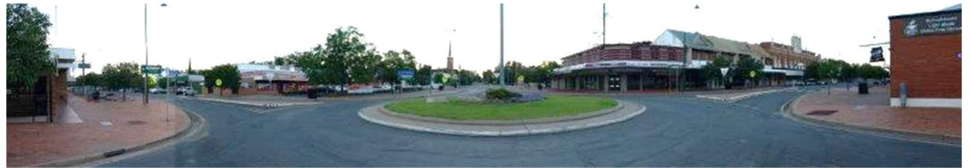
Oxley Hwy/Dubbo St Roundabout (needs to be focal point and provide navigation without clutter/safety issues -see Masterplan)
