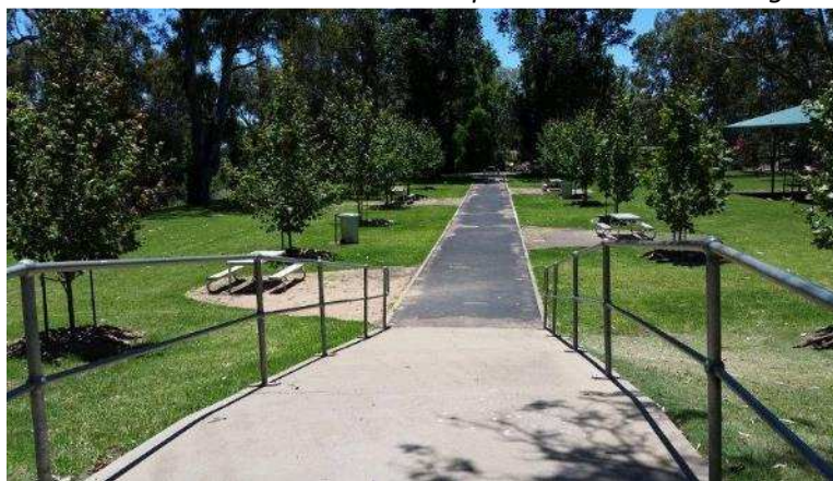
Repair pathway / accessible entries to seating areas
