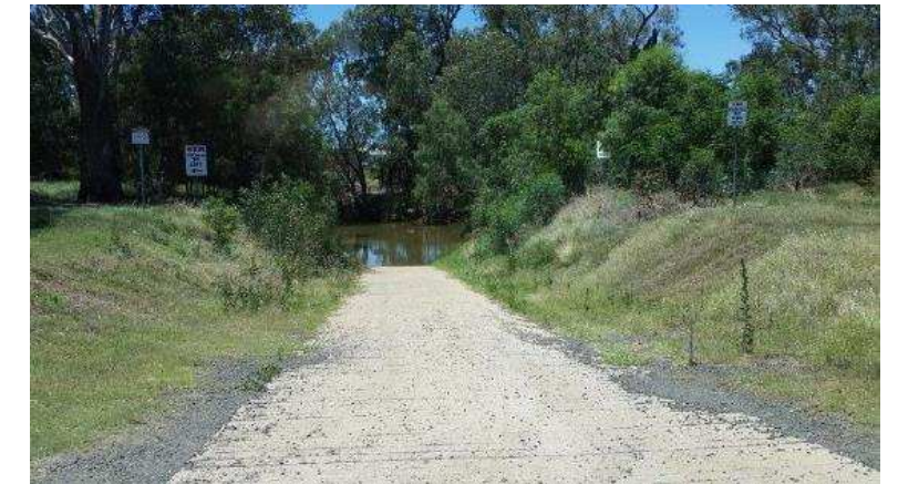
Weir (needs signage/information for visitors)
