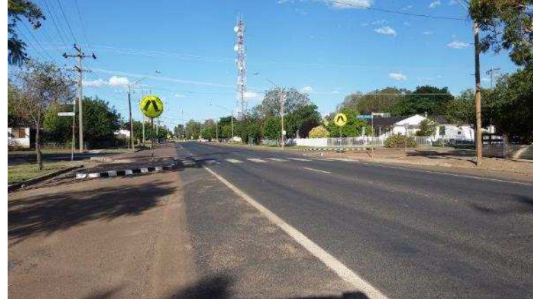
Oxley Hwy/ Burton St – pedestrian crossing (repaint and widen blisters)
