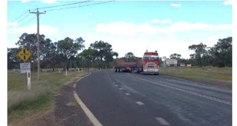
Industrial Bypass intersection (needs signage to camping/future slip lane)
