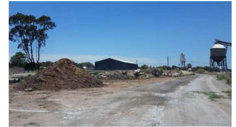
Industrial Area – Silo Road (clean up waste materials)
