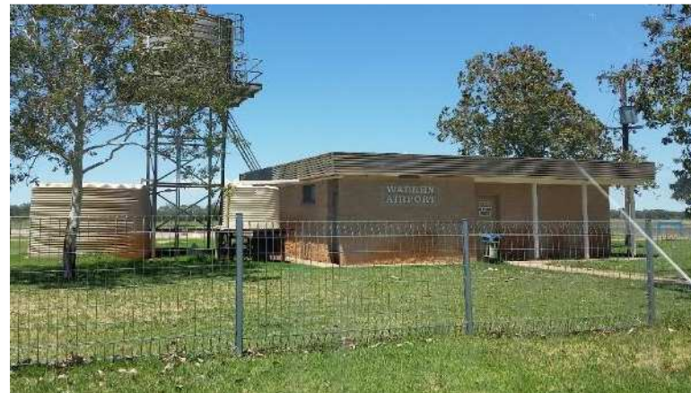
Warren Airport (water to be extended/runway repairs/committee)
