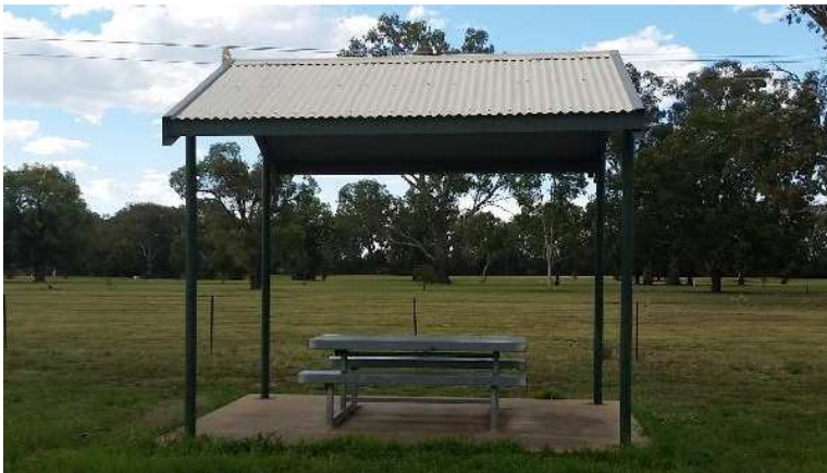
Oxley Hwy Rest Area (south-west) (accessibility upgrades long term)
