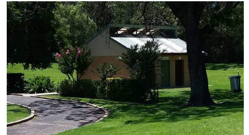
Toilet block (check accessibility / signage)
