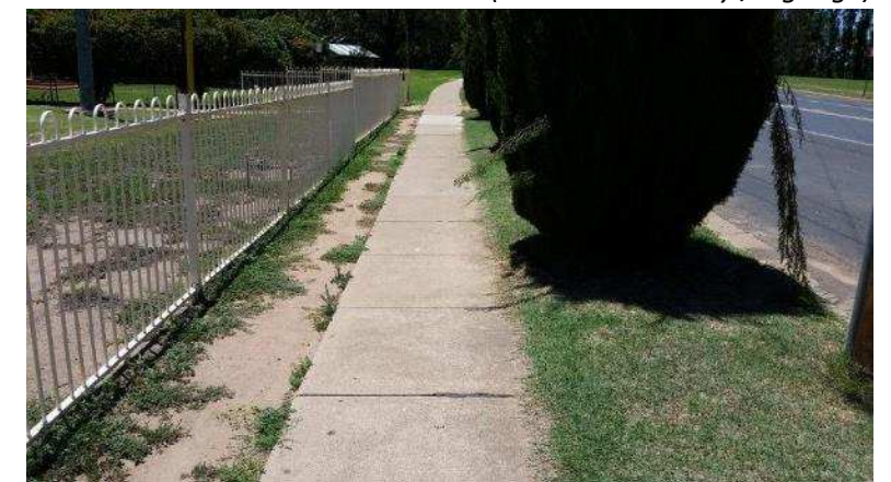
Path along Oxley Hwy to Macquarie Park (requires widening)
