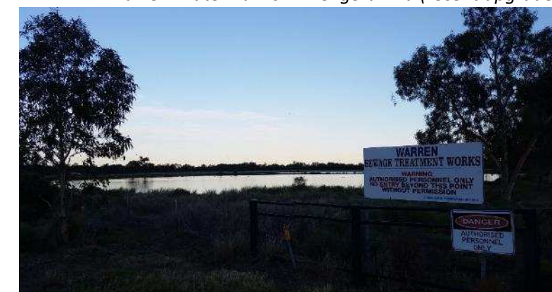
Sewage Treatment Works – Oxley Hwy north-east (water re-use opp.)
