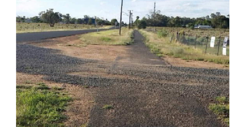
Rotary Centennial shared path near Water Tanks (maintenance/repair)
