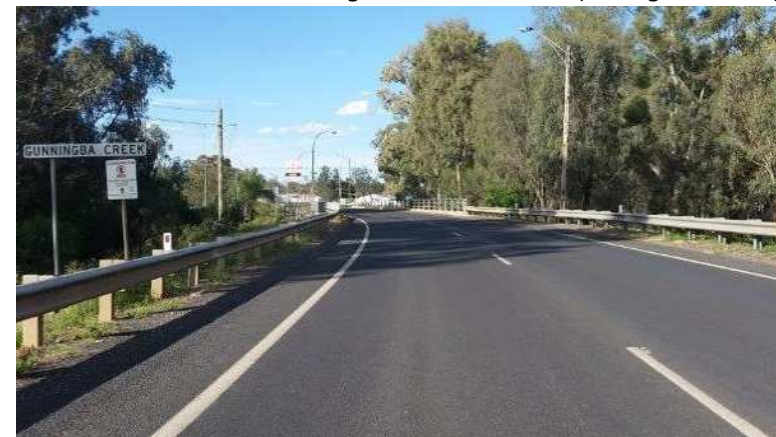
Gunningbar Creek Bridge (review shared path width)
