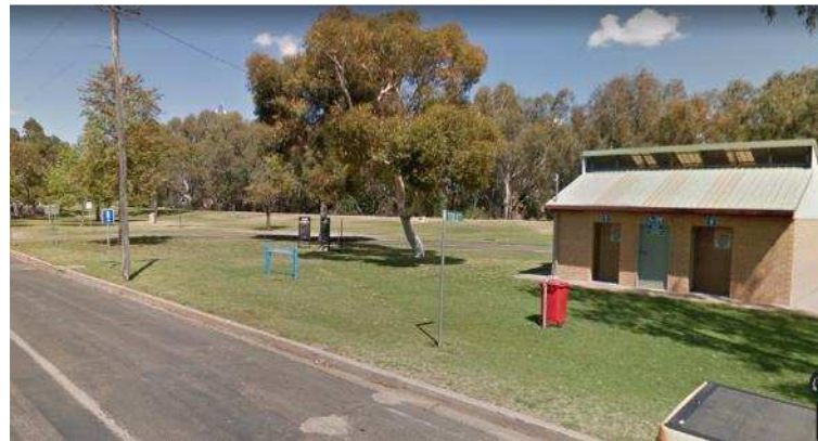
Oxley Park Rest Area (improve driveway and access)(Source: Google)
