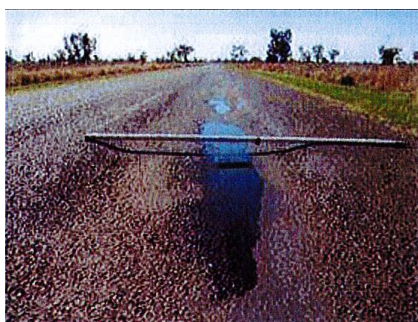
Rutting in wheel paths
