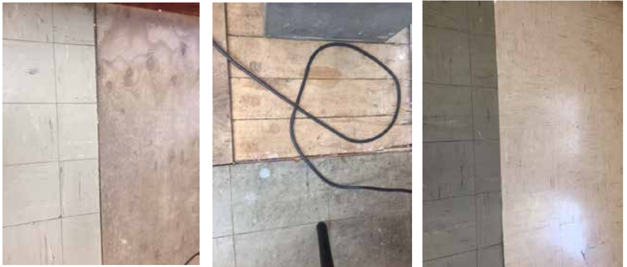
Three sections of the flooring at the Warren Visitor Information Centre
