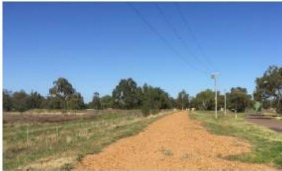
Existing levee bank – Udora Road
