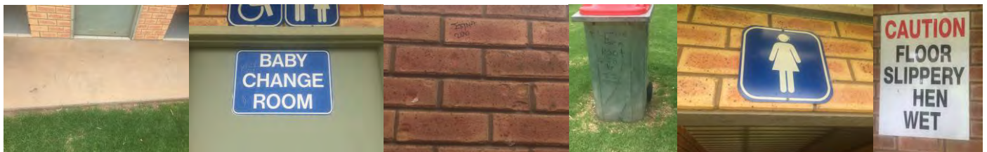
Graffiti on footpath/wall/ bin and various damaged signs
