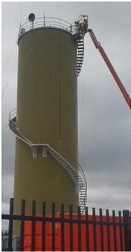
The \$750,000 Nevertire Reservoir refurbishment program is progressing with the contractor recently completing an external washdown, spot priming and the installation of new handrails on the top of the 21-metre-high reservoir.
